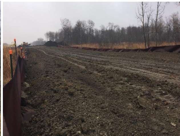
740 + 101 Ramp built over wetland crossings SK 847 an SK 849
