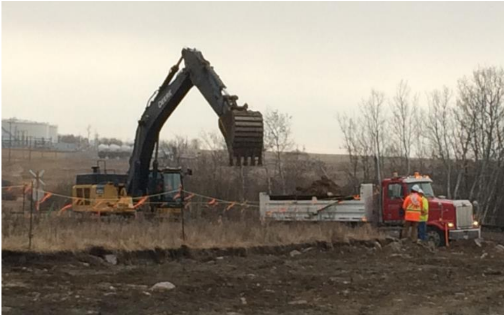
805 + 612 Digging track bore pit west side of the tracks at Pipestone Creek
