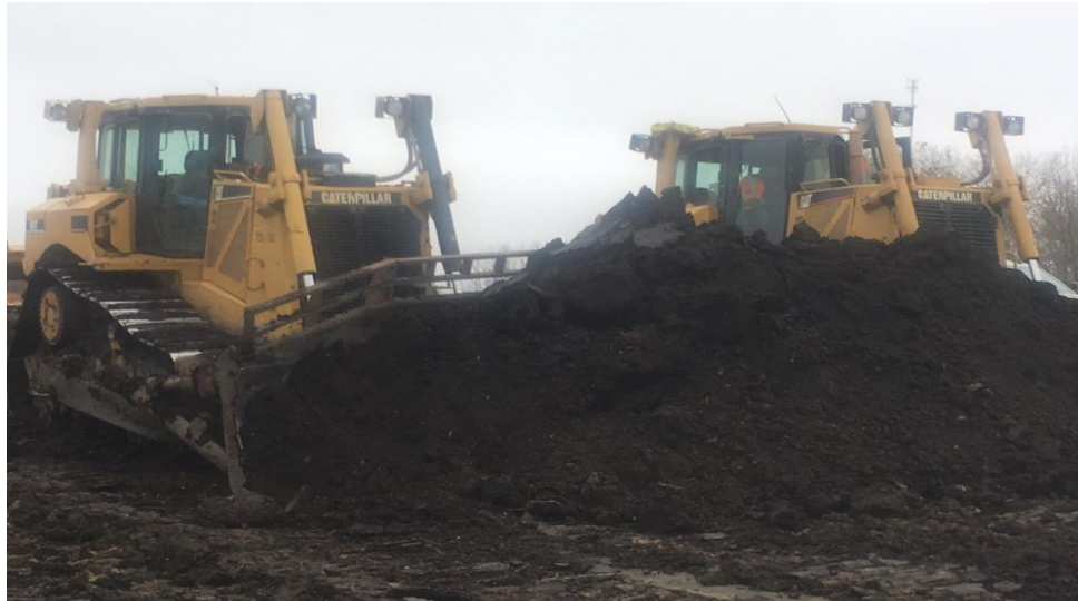
784 + 842 Dozers tandem pushing Stripping to windrow
