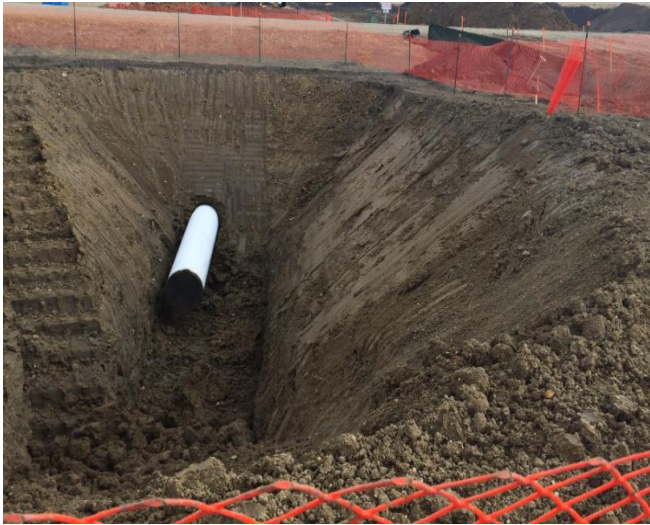
748 + 737 Bore pit excavation for road crossing
