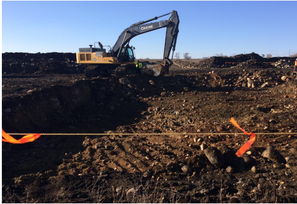
805 + 612 Track bore pit west side of the Pipestone Creek
