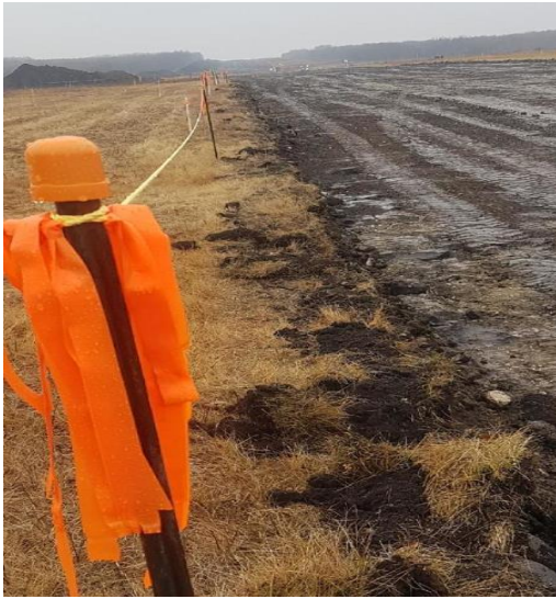
785 + 051 Stony Creek Area of interest roped off and equipment moving top stripped topsoil
