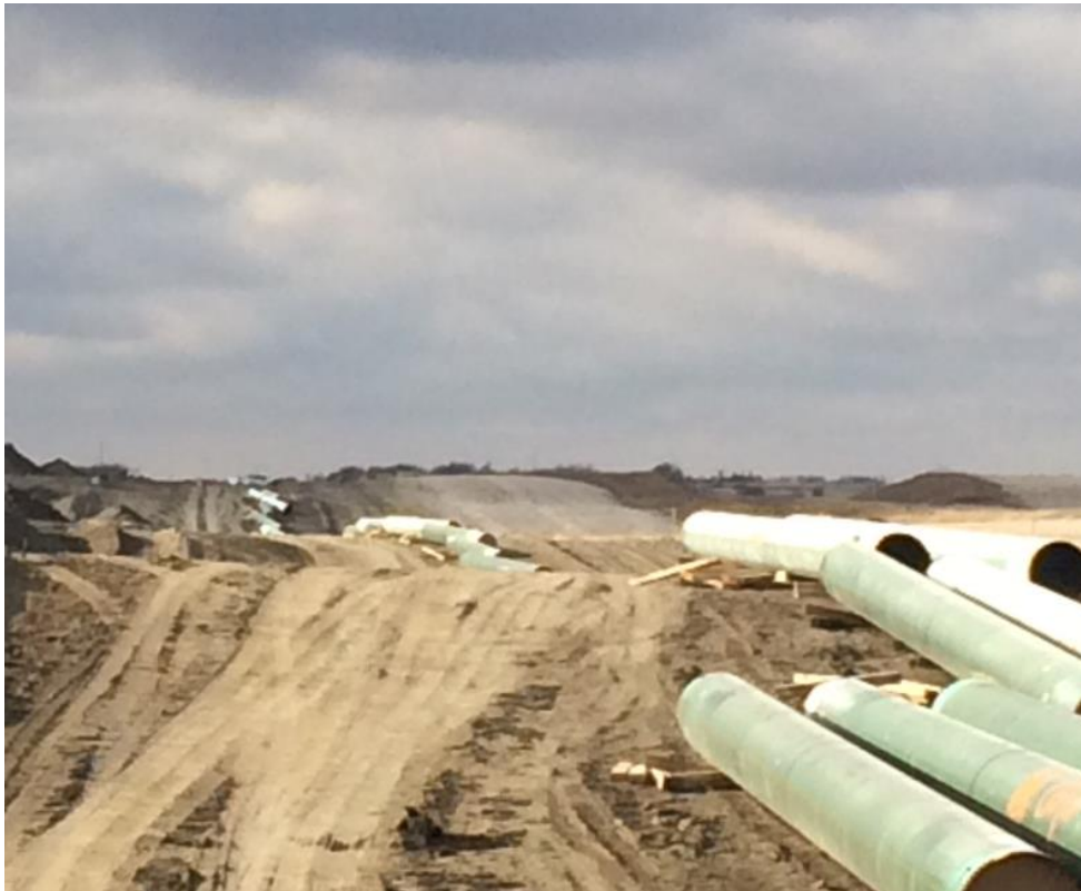
691 + 580 Pipe strung along the right of way
