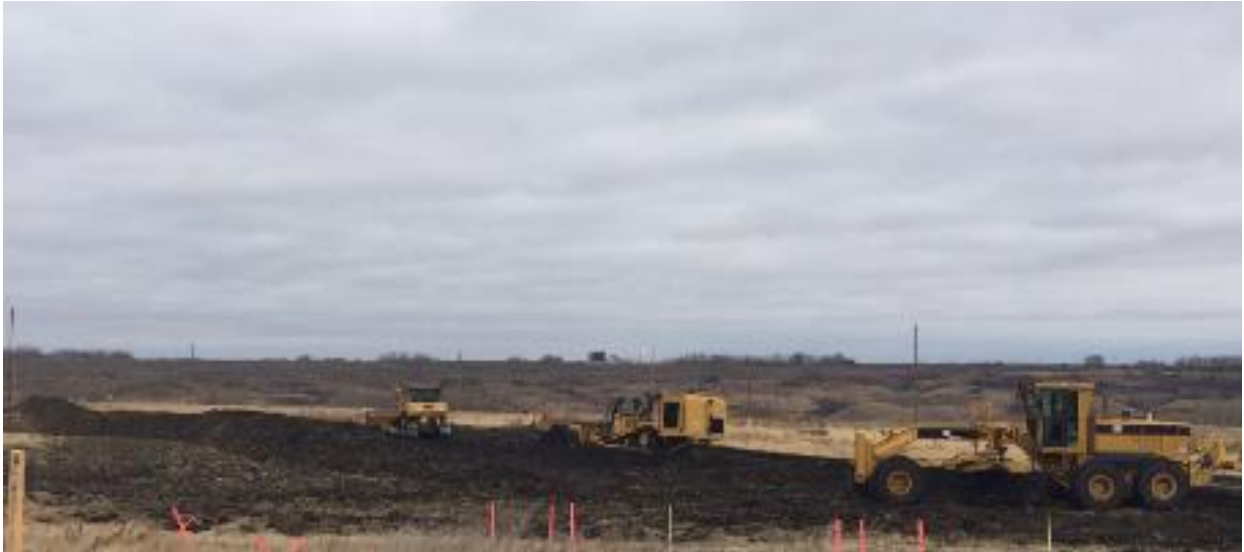
800 +902 Power dozers stripping topsoil
