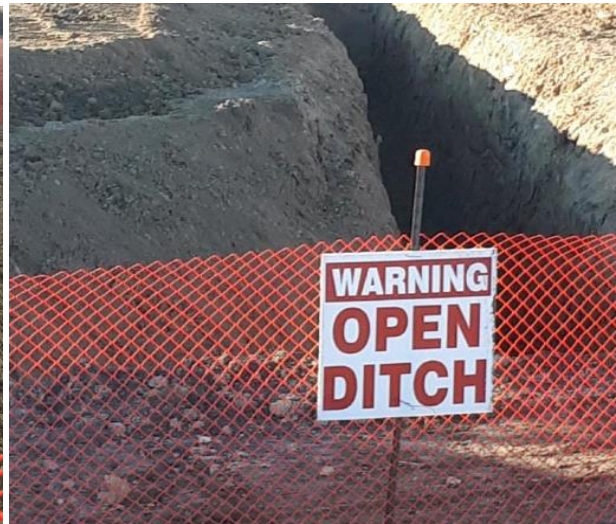
691 + 580 Bore bay and tail ditch excavation
