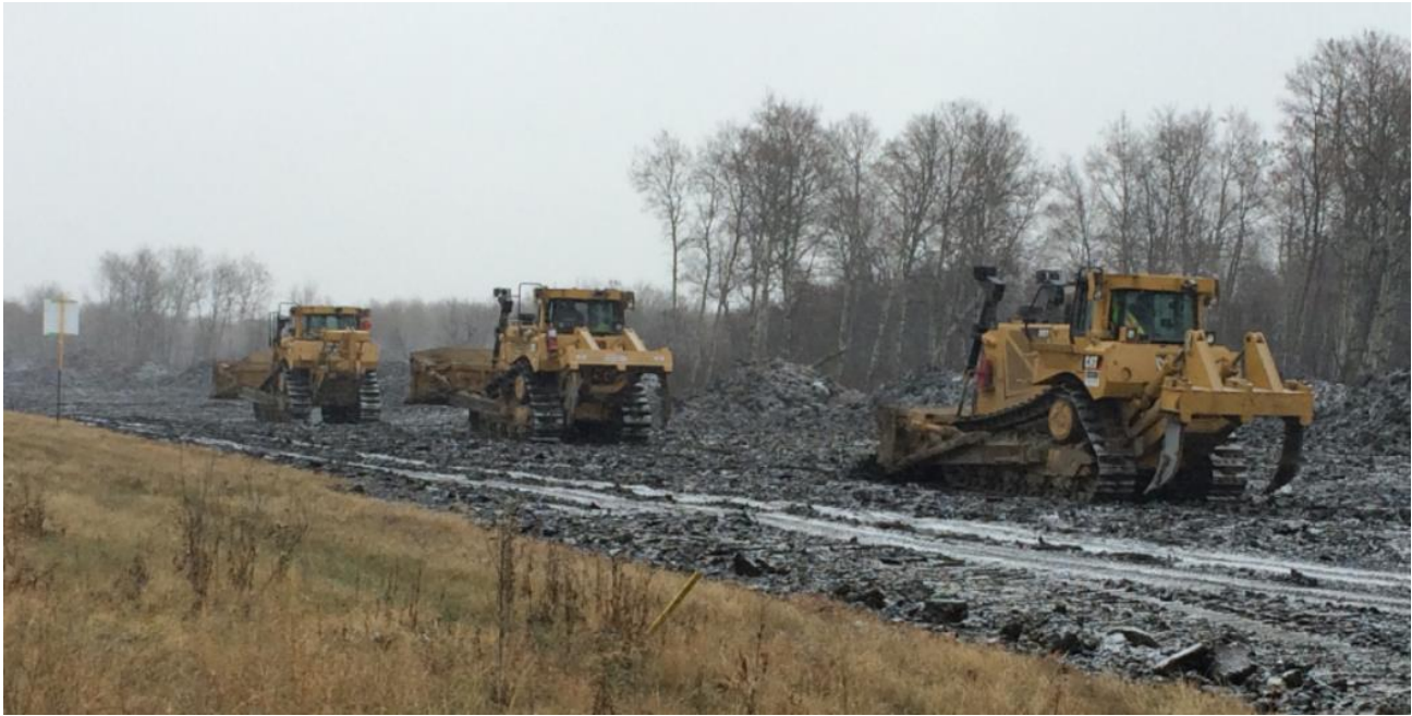
741 + 779 Dozers travelling on right of way to work location
